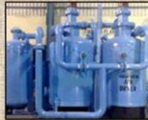
HOC/ No Purge Loss Air Dryer
