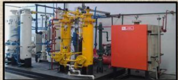
B. NE_UN Nitrogen Generator Purity: < 3 PPM
